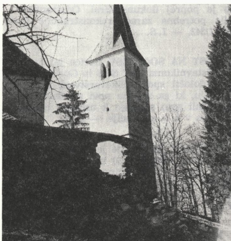
Sl. 7 Krtina, poskodovano obzidje protiturškega obzidja Fig. 7 Krtina, The damaged walls, built against the Turks
