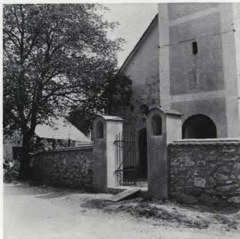
Sl. 132 Zavogljje – pokopališki zid pred in po obnovi Fig. 132 Zavogljje – the cemetery wall before and after renewal
