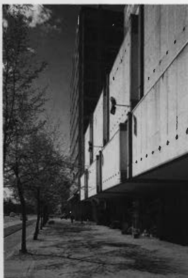
Department store ... "It is a modular layout of the so-called additive architecture, created with ferroconcrete frames with interpolated cubic bodies."
