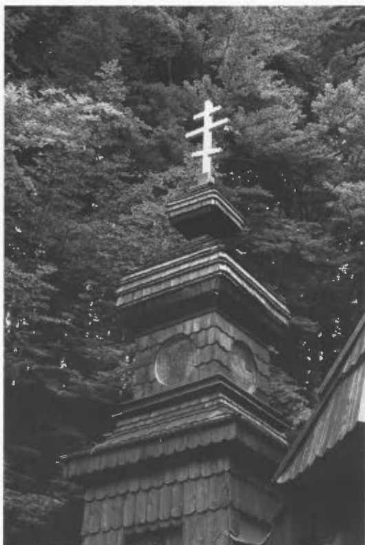
Bell-tower of the chapel. "The shingles of various sizes for the bulbous towers had to be manufactured manually..." .....
