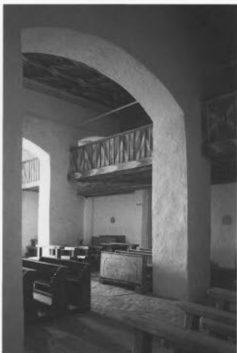
View of the renovated wooden choir. "Therefore the decision to perform the reconstruction of the entire ceiling was taken, with the exception of the choir banister and the ceiling above the choir..."
